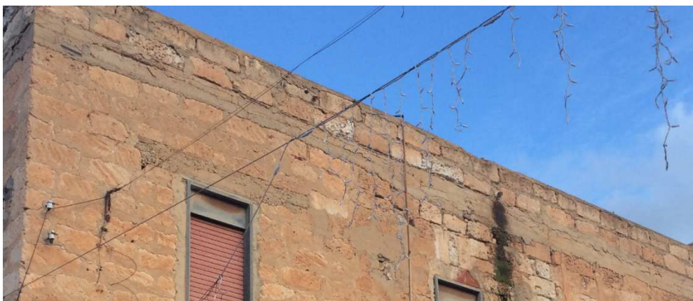
Fig. 14. RC curbs in limestone masonry buildings.
