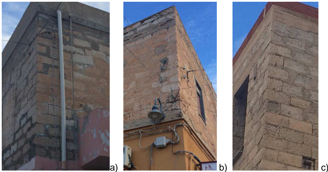
Fig. 16. Effectiveness of corner clumping of buildings. a-b) Limestone masonry; c) Concrete block masonry.
