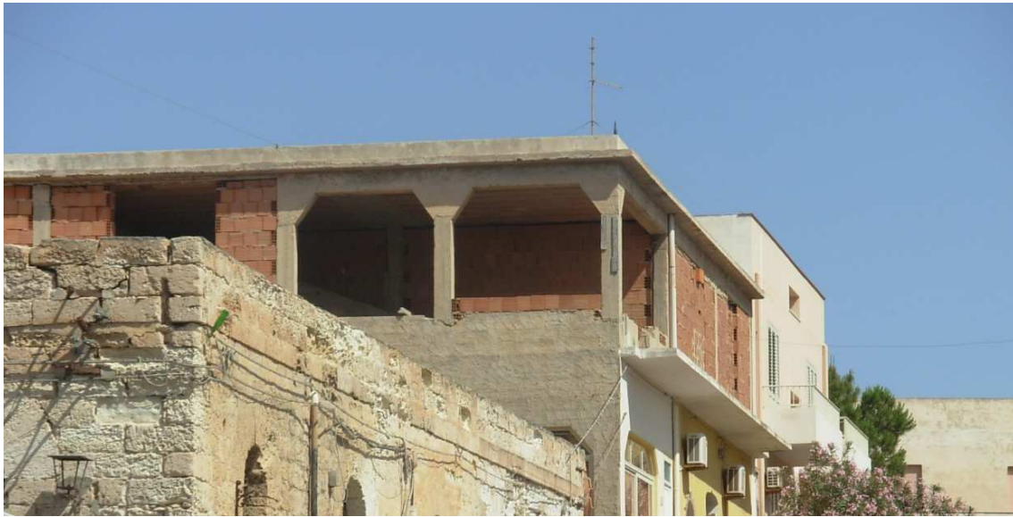
Fig. 18. RC building with frames designed only for gravity loads.
